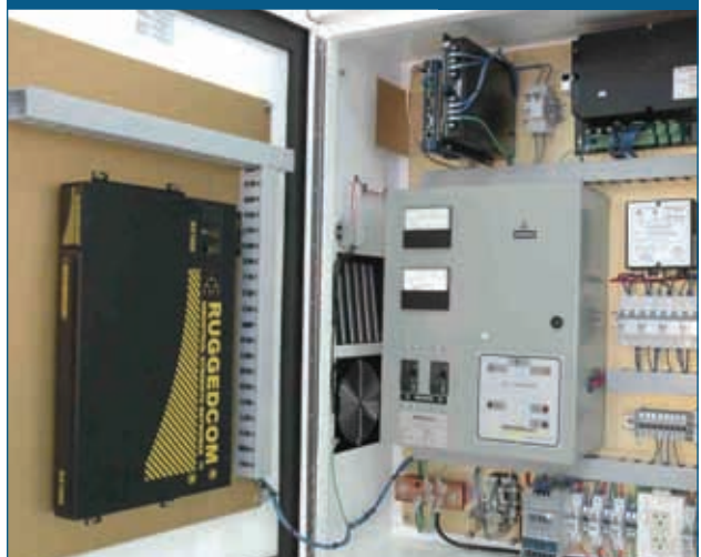
Figure 2. Cooling a panel with an air-to-air heat exchanger avoids corrosion and dirt buildup that can wreck electronics.
